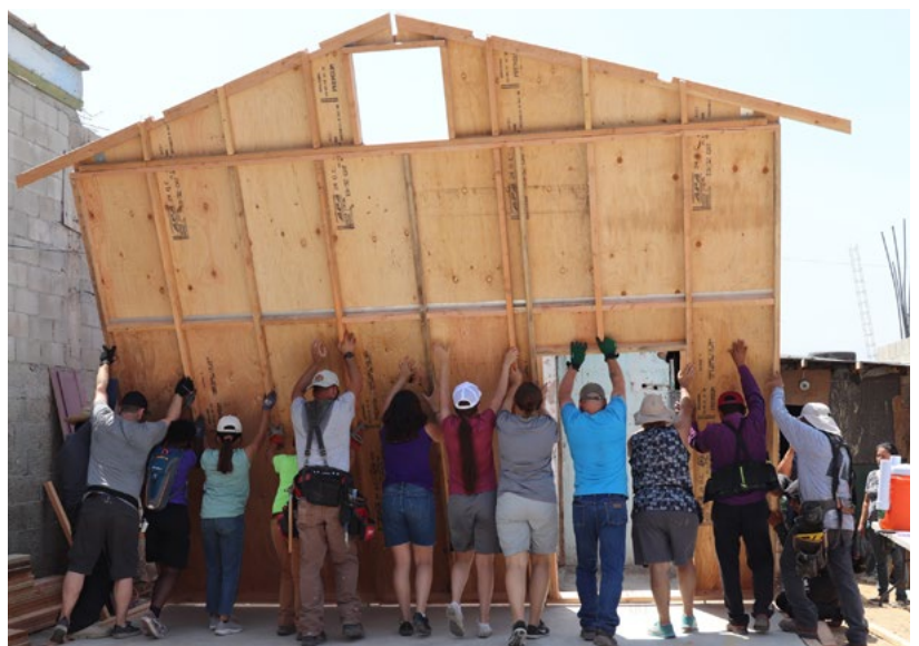
Raising the first wall
